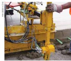
**3:** As the insertion process is started, the vibration will be turned on and the hydraulic cylinder will begin to insert the bar. The operator simply holds or guides the handle on the inserter to keep it stationary with the side of the slab as the paver continues to move forward.
