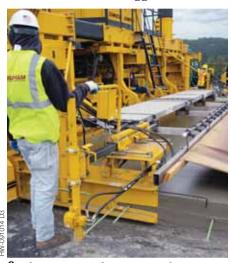
**6:** The operator then moves the inserter apparatus to the forward or home position with the attached handle and the process can begin again.
