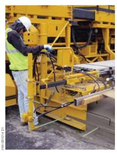
2: The operator places the tie bar to be inserted into the device ready for insertion and begins to monitor the distance gauge rod mounted to the inserter. Once the paver has advanced forward to the point the gauge rod is aligned with the previously inserted side bar, the operator activates the "Start Insertion" toggle switch.
