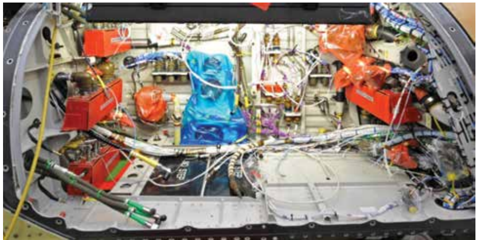
Figure 2: Typical Cable Installation in an Airframe
