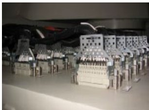
Figure II- 9.3 Han® EE and Han® ESS mounting panel
