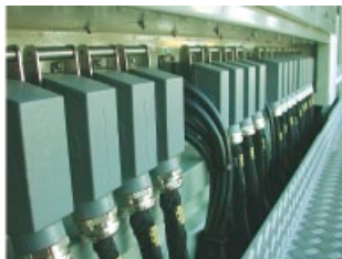
Figure II- 9.2 Han® B with central interlock mecha- nism, used for a current converter
