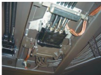
Figure II- 3.2 Entire view of motor connector mounted on vehicle
