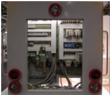
Figure VI- 6.3 Front of vehicle with opened electrical cabinet
