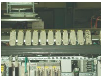
Figure II- 11.2 HARTING connectors used as the interface to the electrical cabinet
