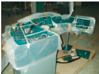
Figure II- 5.2 Driver controls before final installation
