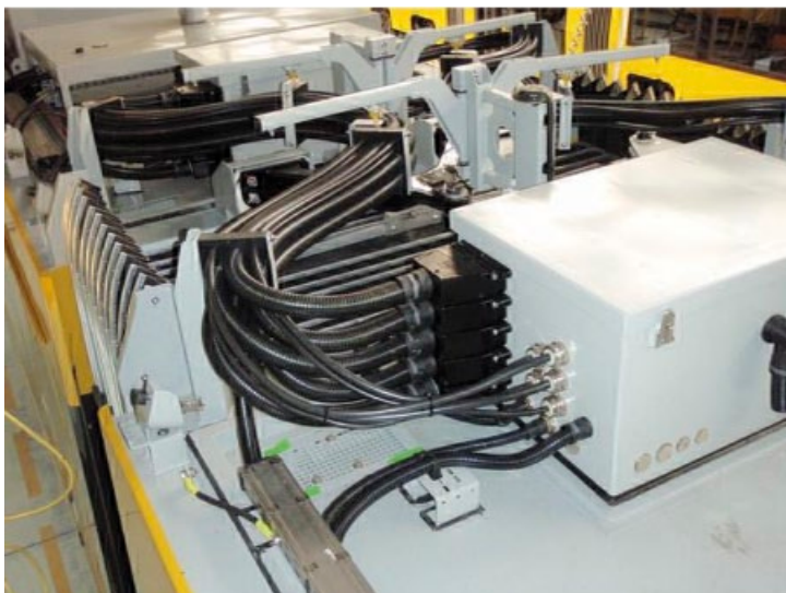
Figure VI- 2.5 Wagon coupling installed on roof
