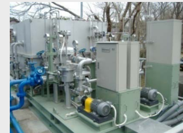
Ozone micro-bubble wastewater reclamation system Demonstration system at Ikenokawa Sewage Treatment Plant
