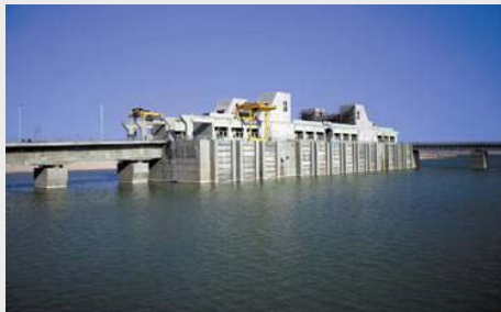
Supplied a large water pump for irrigation to Egypt.
