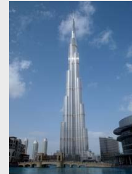
Supplied air-conditioning equipment for the world's tallest building in the UAE.
