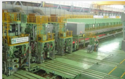
Developed and delivered hot rolling mill control system for Dongbu Steel Co., Ltd., South Korea
