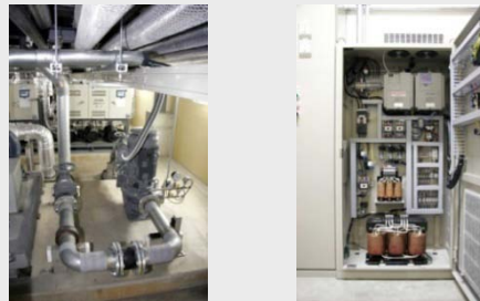
Micro hydroelectric power generation using air-conditioning cooling water and power grid control
