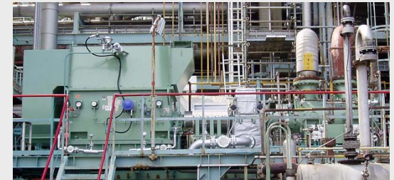
Conversion of compressor drive of existing steam turbine drive to motor-drive in petrochemical plant
