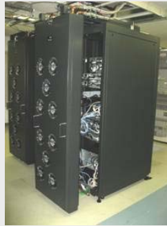
Data center energy-saving air-conditioning system
