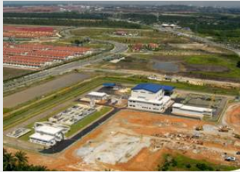
Installed Pegasus* system in sewage water treatment plants in Malaysia
