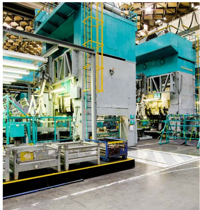
Monitoring of hydraulics on a press
