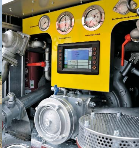
ecomatmobile in a fire engine: The PDM dialogue module visualises the state of the fire water pump system.
