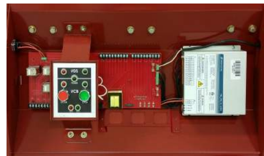
Control Module / Control Circuits (Front Panel Removed)
