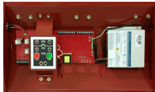
Control Module / Control Circuits (Front Panel Removed)
