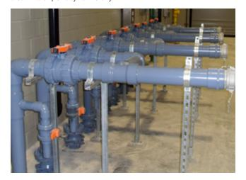
Robert Dragisic, Regional Sales Manager for IPEX USA, worked with the contractors for the pre-treatment portion of the project that was designed to eliminate the radium from the ground water. Products supplied included Xirtec® 140 PVC 80, Corzan® CPVC Piping, VXE Ball Valves in PVC & CPVC, SXE Ball Check Valves
