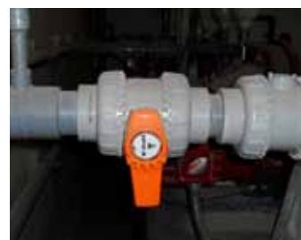
IPEX manual VXE, VX and electric actuated VKD Series Ball Valves were used throughout the facility to control flow as needed.
