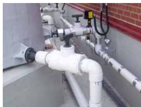
IPEX double containment ball valves were used.
