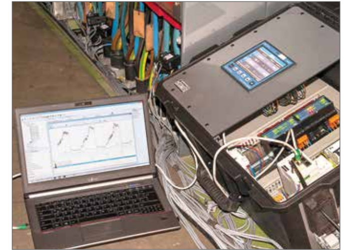
Image 10: Thanks to the open interfaces, the mobile measuring box offers numerous possibilities for evaluation and documentation. Here, a load curve is visible directly on the Notebook.
