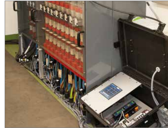
Image 9: The mobile measuring box next to an outgoing section. The split-core current transformers can be fitted and disassembled at the line connection without intervention. That makes mobile use possible in the first place.
