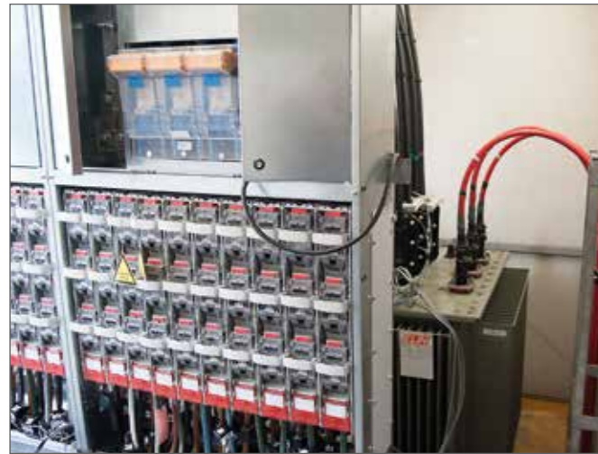
Image 7: The converters are installed at the outlets and at the supply lines from the transformer. This provides a complete picture of the overall situation.
