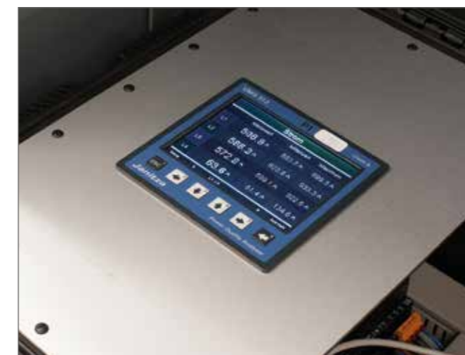
Image 4: As the measured value memory shows, the monitored outlet is well utilised. The nominal current is 1000A, phase L2 was partially loaded with 933 A.
