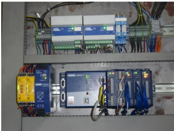
Fig. 3: The installation situation of the automation system
