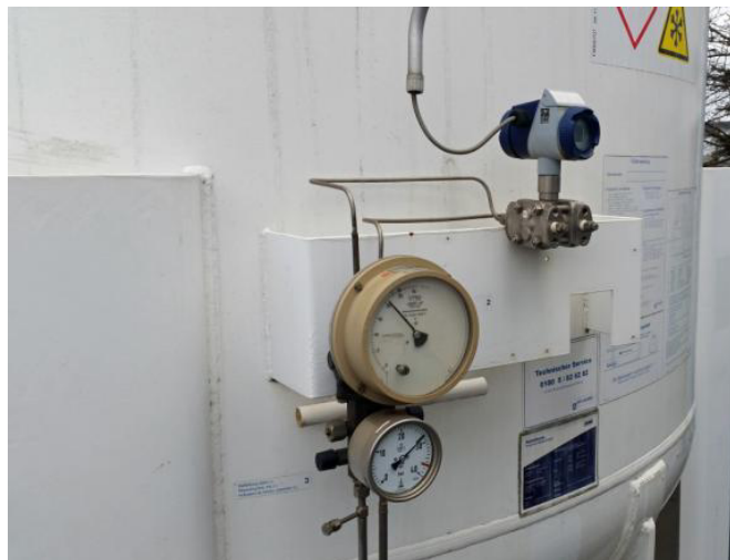
Fig. 2: Installation situation on the tank system
