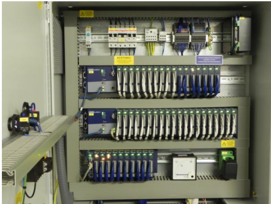
Figure 1: Control cabinet with the JUMO mTRON T automation system
