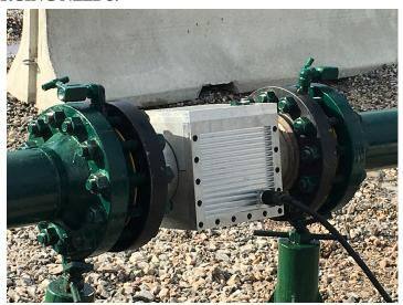
Lightning Master's innovative  $\underline{I}_n$ - $\underline{P}_i$ pe  $\underline{T}_i$ urbine  $\underline{G}_i$ enerator (IPTG) system is designed to provide electricity at isolated locations lacking commercial power. It generates power using the flow of gas through the pipeline without combustion of fossil fuels.
