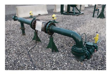
Lightning Master's innovative IPTG system is designed to provide electricity at remote locations lacking commercial power. It generates power using the flow of natural gas through the pipeline without combustion of fossil fuels.
