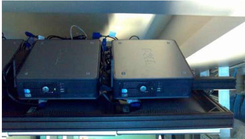
Fig. 4. Small computers can fit behind the display tile, simplifying cabling and hiding the computers.
