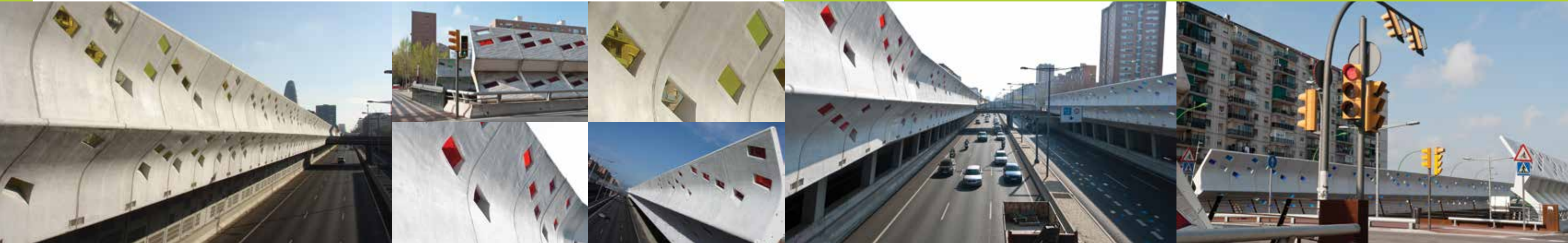
Images: Spanish architects, Arquitectura Blanca, used over 16 tonnes of Polycasa cast acrylic in the construction of a 2km sound barrier wall along Gran Via de les Corts Catalanes in Barcelona. Areas of cast sheets in 12 different colours were inserted along the full length of the barrier wall producing a rainbow effect along the route. The material was supplied by Polycasa's customer, Comercial Arteplástica. The project was developed in two phases, the first in 2006 and the second in 2011. The cast acrylic sheets were manufactured by Polycasa in Barcelona using MMA supplied by Lucite International.
