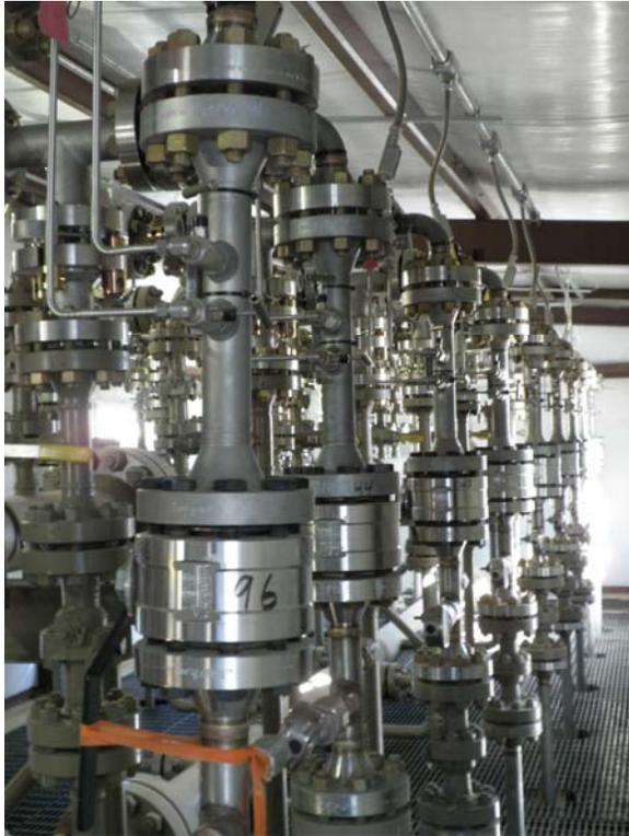
Figure 2: Installed V-Cone Flowmeters
