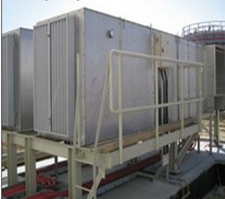
The substation at Kuwait Int. Airport housing the gensets/loadbanks.
