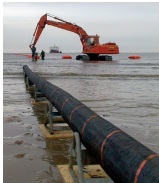
Installation of power cable, Horns Rev 1, in Denmark.
