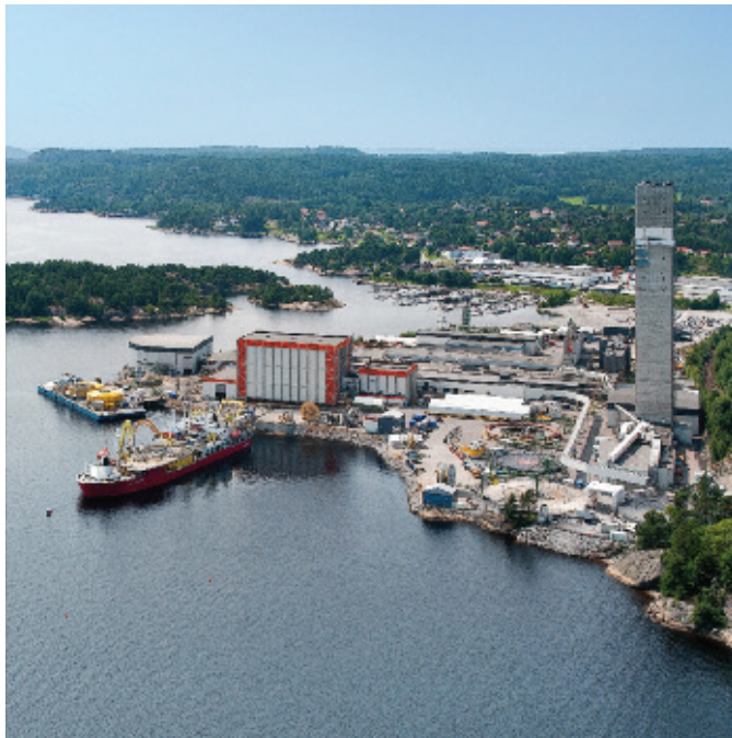
The tower in Nexans Halden factory has two XLPE lines for parallel production.
