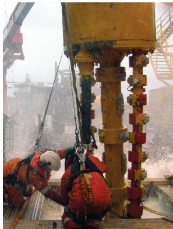
Installation of subsea junction box.
