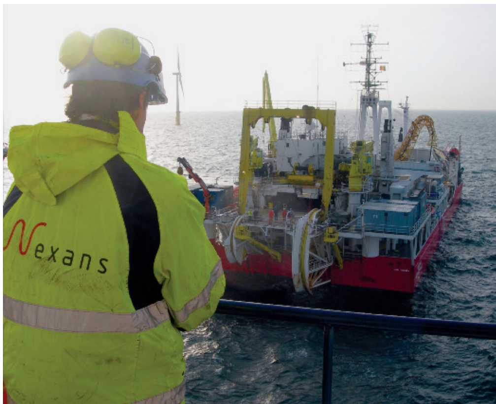
Installation of the Belwind project was carried out with Nexans' cable laying vessel C/S Nexans Skagerrak. Nexans' Capjet system was used for trenching the cable that was delivered in the summer of 2010.
