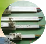
LV building cables
