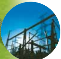
HV/MV joints and terminations
