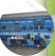
Control room cables
