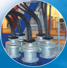
Auxilliary equipment and systems
