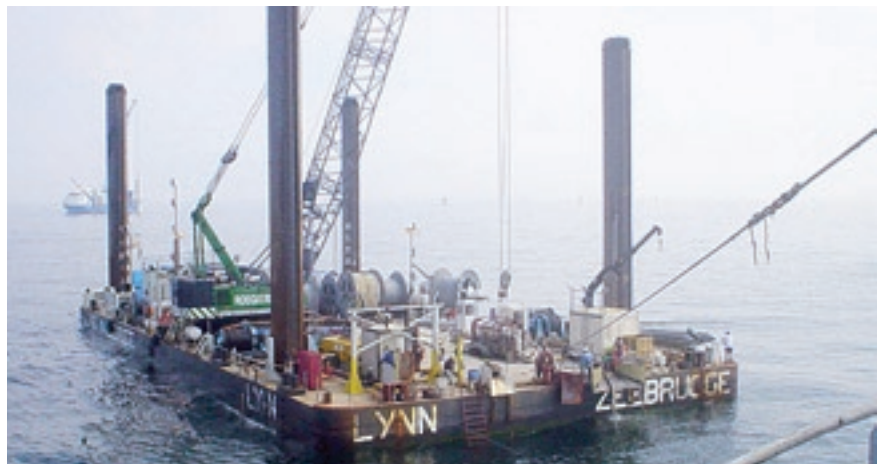
Cable laying within an offshore windfarm
