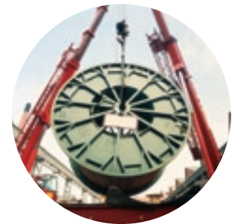
Lifting a submarine power cable drum for Abu Dhabi
