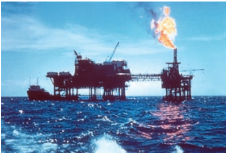
Offshore production platform in Indonesia, with power supply through a submarine cable
