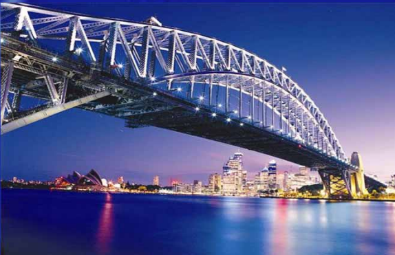
Bridge and Building Monitoring
