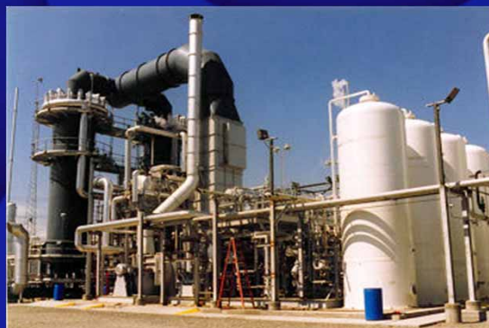
Steam Plant Monitoring
