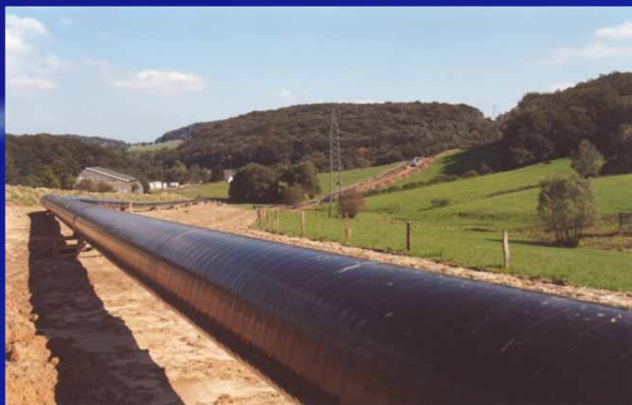
Oil, Water, Gas Pipeline Monitoring
