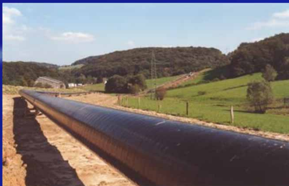
Oil and Gas Pipeline Monitoring
