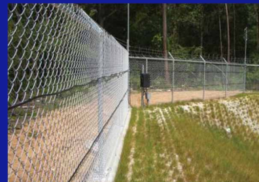
Border Security Monitoring
