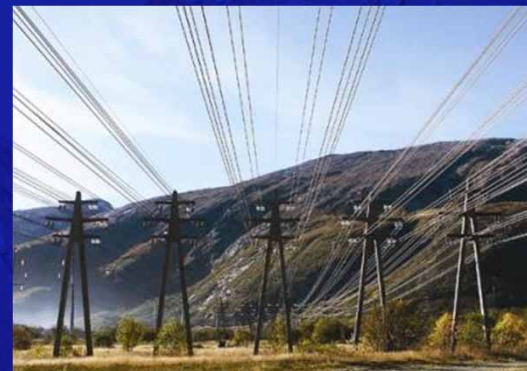
Power Line Monitoring
