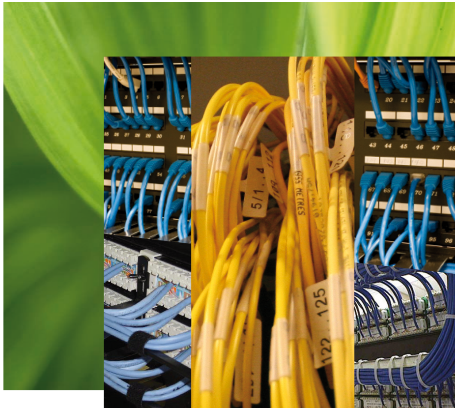
You quickly get a survey over exactly which distribution frames and cables the connections must go through, all the way from the main distribution frame to the individual user plugs
