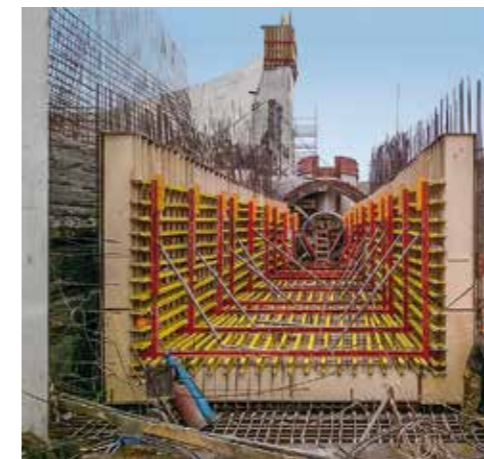
The 3D tunnel formwork construction on a VARIOKIT system basis allowed the dimensionally-accurate realization of the transition from square-shaped to circular discharge structure cross-sections.
