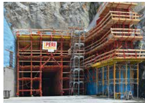
An integral part of the PERI solution was the formwork carriage and wall formwork for constructing the two intake structures with up to 3 m thick reinforced concrete slabs.
