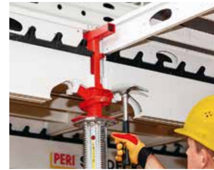
One blow of the hammer releases the drophead; in the process, the formwork is lowered by 6 cm. Main beams and panels can then be struck.
