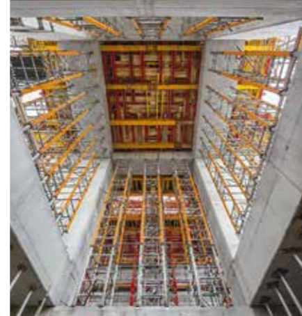
Modular supporting systems made it possible to easily adapt to the complex building structure.
