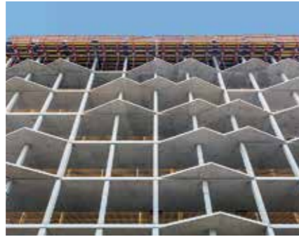
VARIODECK and PROKIT guaranteed a high level of safety during construction of the residential towers complete with triangular oriels.
