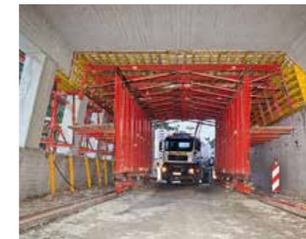
With this slab formwork carriage, a 3.00 m wide and 4.50 m high drive-through opening ensured unobstructed site traffic operations.
