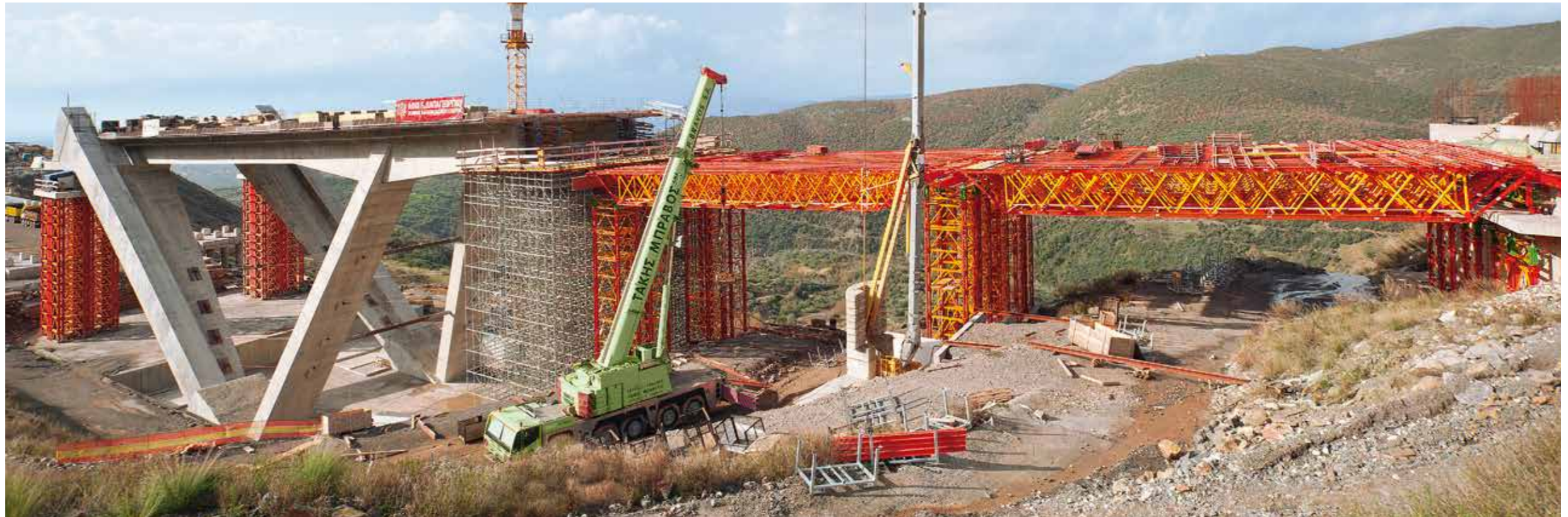
These 23,60 m high heavy-duty shoring towers each carry loads of over 200t. 10 m high tower sections were pre-assembled which accelerated the construction process.
