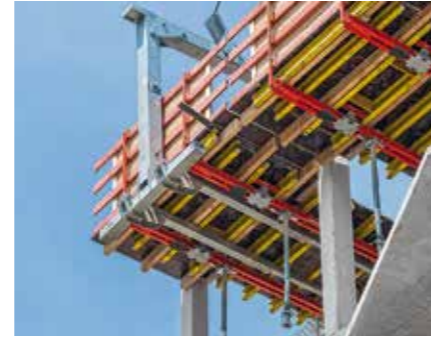
The VARIODECK Edge Tables were moved as large-sized units including guardrails with the help of the PERI Transportation Fork.
