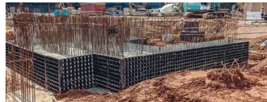
Due to the manageable dimensions of the DUO panels, these are also ideally suited for the construction of foundations.
