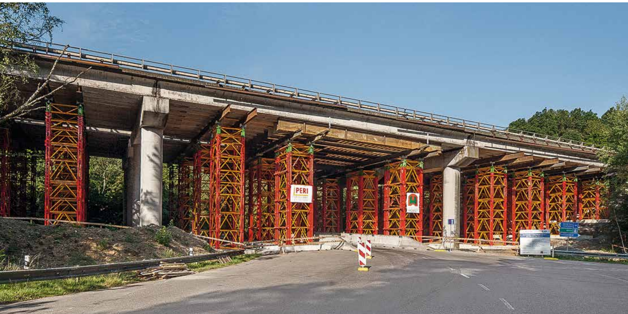
Compatible: the PERI UP Scaffolding System ensured safe access and accelerated the VARIOKIT assembly.
