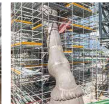
The Modular Scaffolding could be flexibly adapted to suit the organic form in 25 cm increments.
