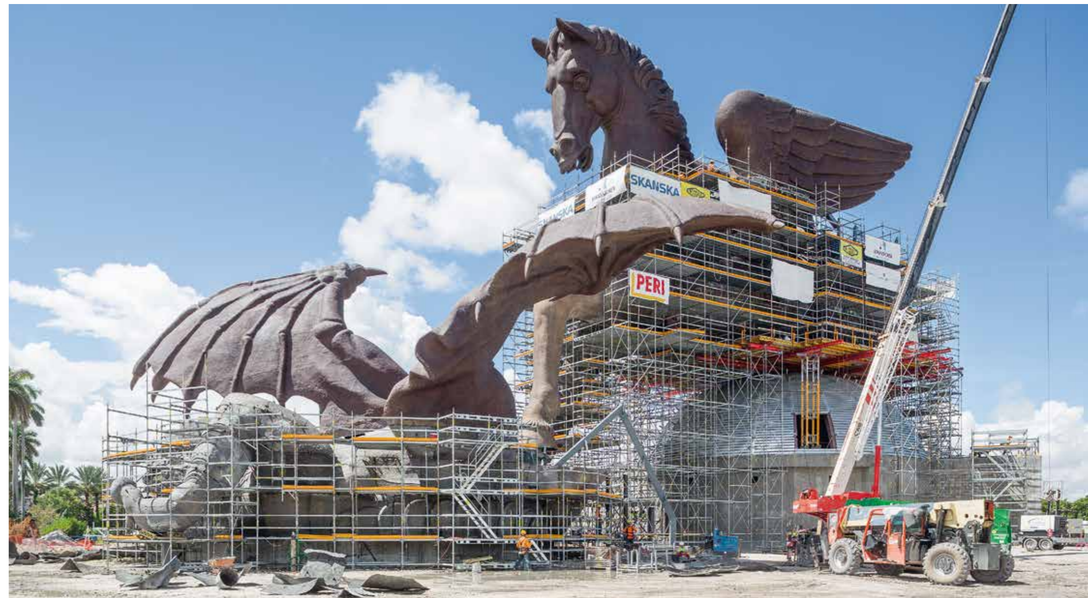
VARIOKIT System Components supplemented the PERI UP Scaffold Solution in particular for the large-span bridging.
