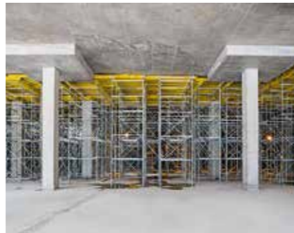
PERI UP shoring towers support the MULTIFLEX Girder Slab Formwork in order to efficiently construct the cast in-situ slab at a height of almost 8 m.
