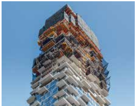
Offset-arranged floors and countless cantilevered balconies required a detailed formwork and enclosure concept.
