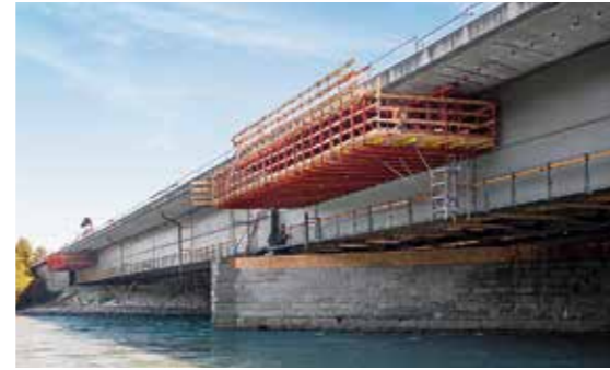
The refurbishment of the 185 m long Inntal Bridge was carried out by two complementary PERI modular construction systems – to a large extent without restricting road traffic.
