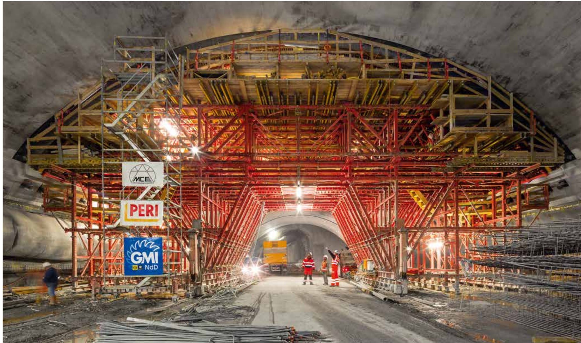
An integral part of the PERI solution was the formwork carriage and wall formwork for constructing the two intake structures with up to 3 m thick reinforced concrete slabs.
