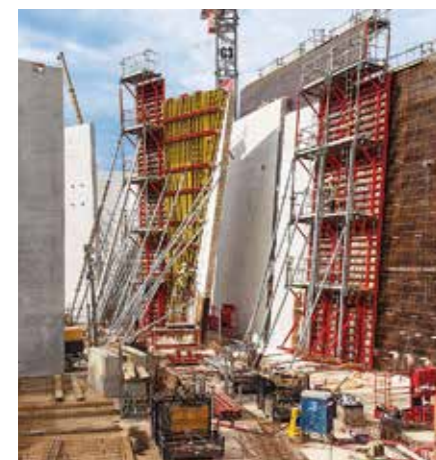
The wall formwork combination using TRIO and VARIO allowed the construction of the 13.50 m high walls with variable inclinations.
