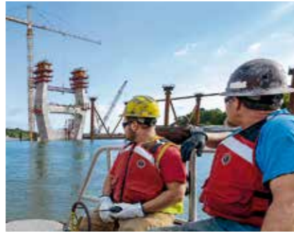
Continuous construction support and a competent planning service: the catwalk featured between the two pylon legs was also an integral part of the PERI complete solution.
