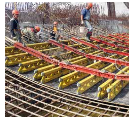
PERI planned and delivered customized solutions for the complex building geometries.
