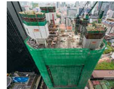
For the RCS enclosure, different materials can be used, e.g. LPS mesh panels, trapezoidal sheeting, multi-layer wooden boards or netting.
