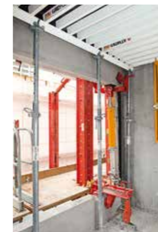
Several RCS Climbing Rails were anchored on the parapets and additionally fixed to the slab.
