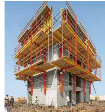
Contractor Azmeel Contracting & Construction Corporation Field Service PERI Saudi Arabia Ltd., Jeddah
