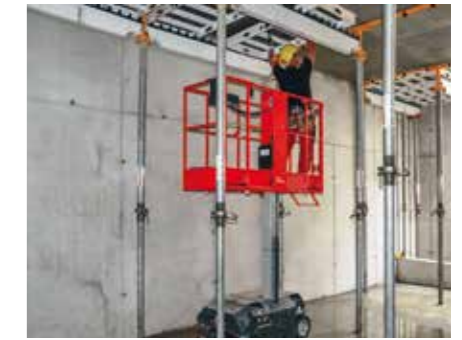
The lifting platform allows safe shuttering and striking operations. It can also be used for reworking tasks or dismantling the shoring construction.
