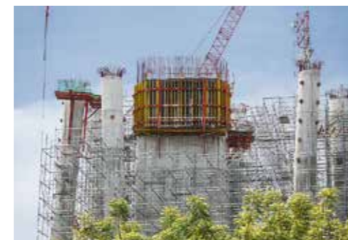
Working scaffold, bracing and shoring rolled into one: PERI UP subsequently followed as birdcage scaffolding within the cycle of the RCS Climbing Formwork.
