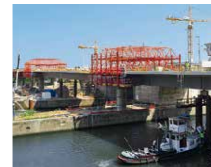
This lock bridge is being constructed with 2 VARIOKIT Composite Formwork Carriages in 13 casting segments using the back-step construction method.
