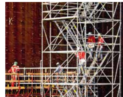
Height adjustments to building openings are carried out by means of short flights of stairs and externally mounted brackets – regardless of the floor height.
