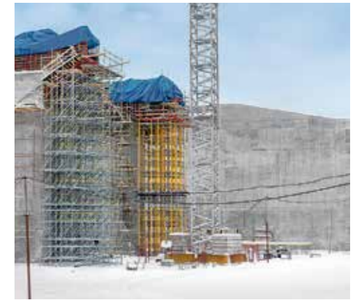
The massive reinforced concrete piers widened out in the head section. MULTIPROP and PERI UP reliably transferred the high loads from great heights into the ground.
