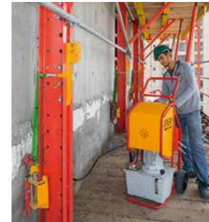
Mobile RCS hydraulic aggregates and cylinders reduced the cost expenditure for crane-independent climbing.
