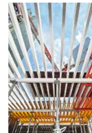
Construction of the floor slabs was carried out with help of GRIDFLEX Girder Grid Slab Formwork system.
