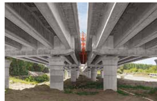
The foreland bridges are supported on 180 cm thick circular columns – here, too, PERI supplied a customized formwork solution.
