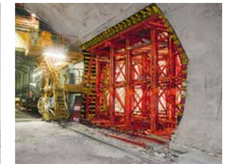
This tunnel formwork carriage on the basis of the VARIOKIT modular system is used for constructing the accessible cross passage between two tunnel tubes.
