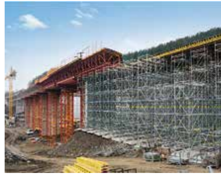
Cost-effective: the PERI bridge formwork concept was based on rentable modular construction systems with standardized components.
