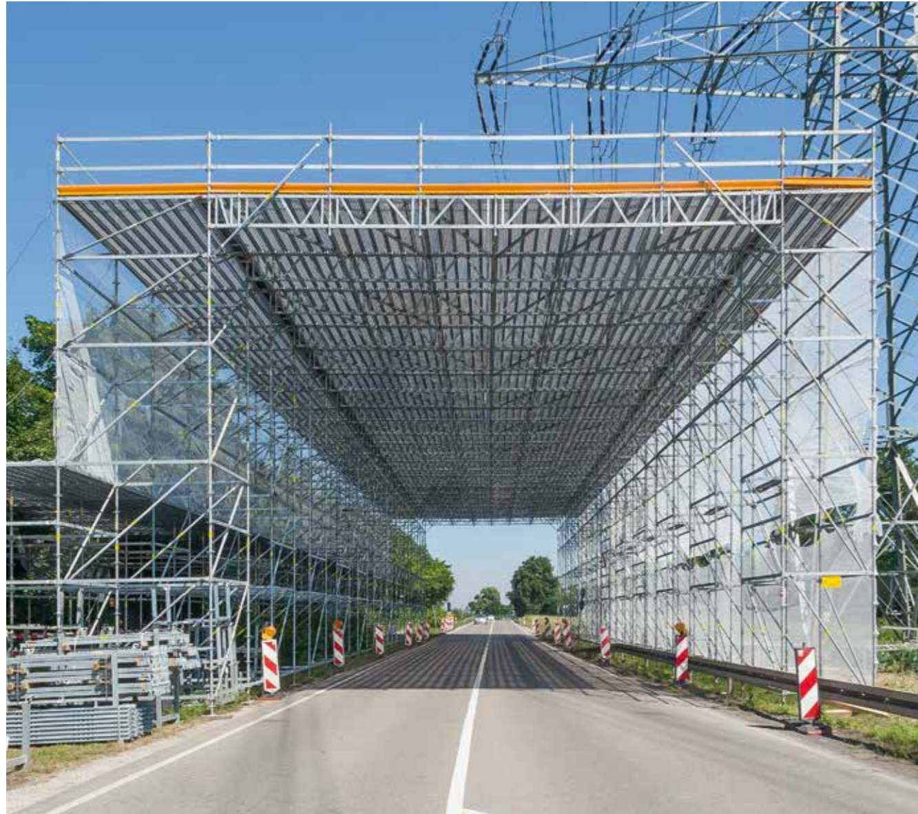
For work carried out on overhead lines, PERI UP protection scaffold comprised of lightweight system components secured the crossings over the public roads.
