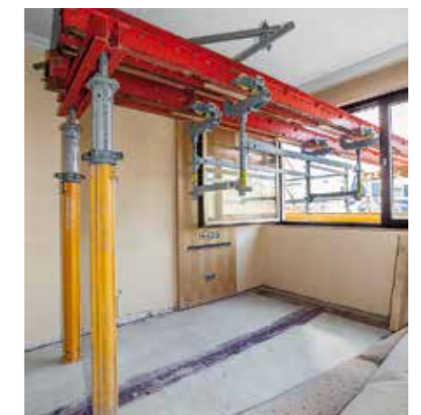
Using RCS Rails and Trolleys from the PERI UP System allowed bulky components to be easily moved through the window openings to the outside.
