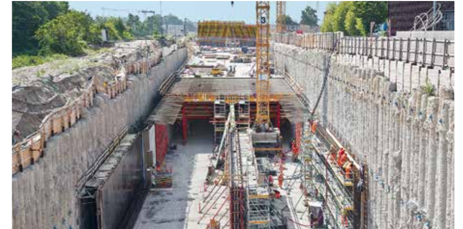
The “Nordhavnsvej – Vej- og Tunnelentreprise” major infrastructure project connects the North Harbour in Copenhagen with the Helsingør motorway. The 620 m long tunnel route runs through a very densely built-up inner city area and also crosses a busy railway line.
