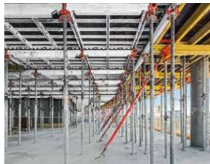
For the two flanking office towers, SKYDECK was supplemented at the slab edges with slab tables.
