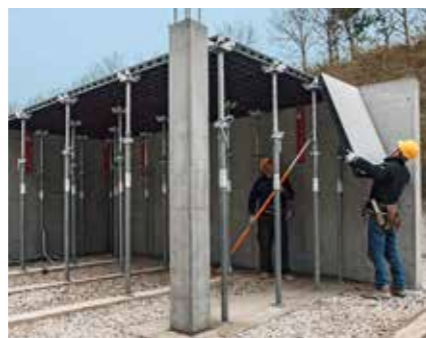
When forming the slab, work is completely carried out from a safe position below; the panels are simply hooked in and then pivoted upwards.
