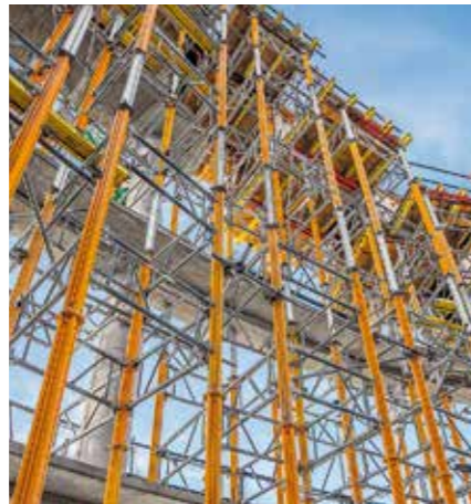
MULTIPROP shoring towers up to 16 m high were used to provide the form-giving load-bearing system for the reinforced concrete edge beams.
