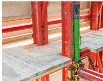
Mobile climbing units lifted the rail-guided RCS Climbing Protection Panel from storey to storey.
