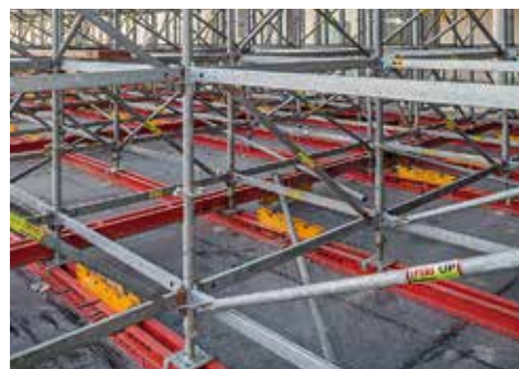
For earthquake-resistant implementation, PERI UP was supported on a load-distributing VARIOKIT construction.
