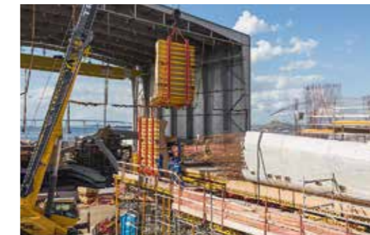
Supported by PERI UP shoring and working scaffolds, as well as a VARIOKIT raised formwork unit, the customised elements could be assembled on-site to form a complete 3D formwork construction.
