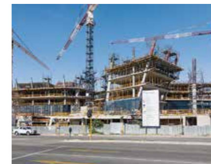
The administration building is characterized by obliquely-arranged building structure and cantilevered slabs.
