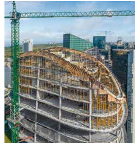
The edge beam construction for the tower finish placed very high requirements on construction operations.
