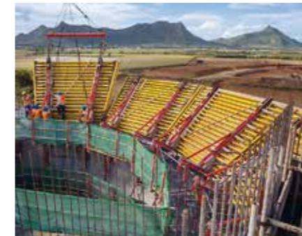
Special suspension points ensured that the formwork elements could easily be lifted into the respective final position with the crane.
