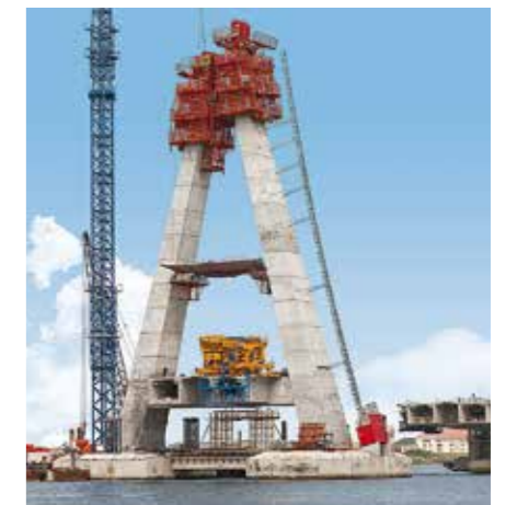
For the construction of this 90 m high pylon, the RCS and ACS climbing systems were combined.
