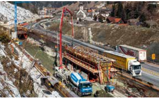
With help of the VARIOKIT Tunnel Formwork solution, 25 m long sections of the tunnel arch could be concreted in regular 4-day cycles.
