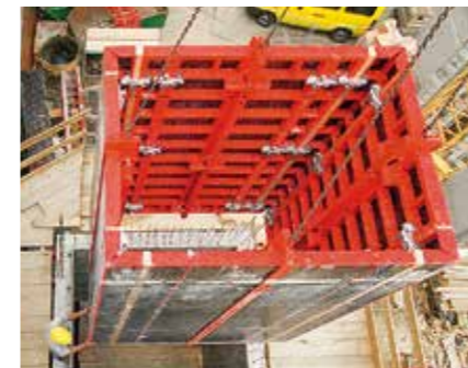
With the TRIO shaft element, complete shaft internal formwork can be moved quickly; the all-round striking clearance is 30 mm.
