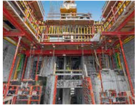
The self-climbing ACS P Platform variant was adapted to suit the central 8 m x 10 m core ground plan while suspended DOMINO elements served for subsequently constructing the intermediate walls.
