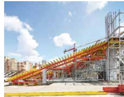
The two modular construction systems, VARIOKIT and PERI UP, formed shape-generating shoring for realizing the inclined grandstand stringers.
