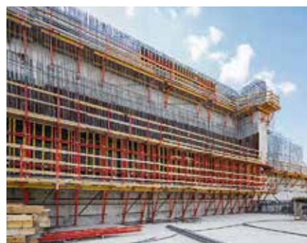
VARIO Formwork, CB Climbing Platforms and PERI UP access technology guarantee easy handling along with a high level of safety.
