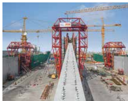
Side walls and centre wall were constructed with the help of three PERI formwork carriages – with a fast working speed and high quality of workmanship.
