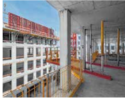
PROKIT provided gap-free enclosure of the building shell slab edges, including the transition area to the cantilevered-mounted RCS MP Landing Platform.
