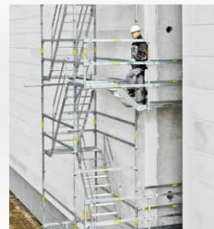
Height adjustments to building openings are carried out by means of short flights of stairs and externally mounted brackets – regardless of the floor height.
