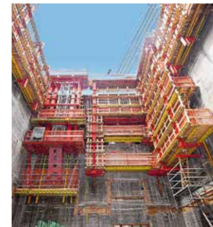
With the ACS self-climbing technology, the concrete placing boom and suspended stair towers can also be moved upwards with any crane assistance.
