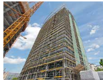
PERI UP Facade Scaffolding allowed fast and safe execution of all reworking operations
