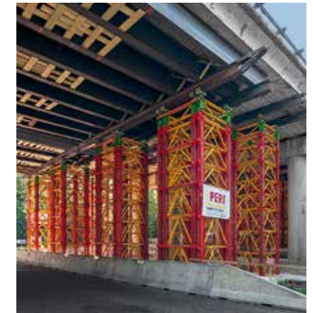
Concentrated: with the help of additional legs, the load-bearing capacity was individually adapted to accommodate the increased load from the carriageway bridging.
