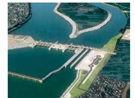
The new Nile barrage is used for water regulation and electricity generation; for ensuring smooth shipping operations, a 120 m long double sluice bridges the 4 m difference in height.
