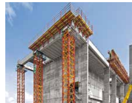
These 23,60 m high heavy-duty shoring towers each carry loads of over 200t. 10 m high tower sections were pre-assembled which accelerated the construction process.
