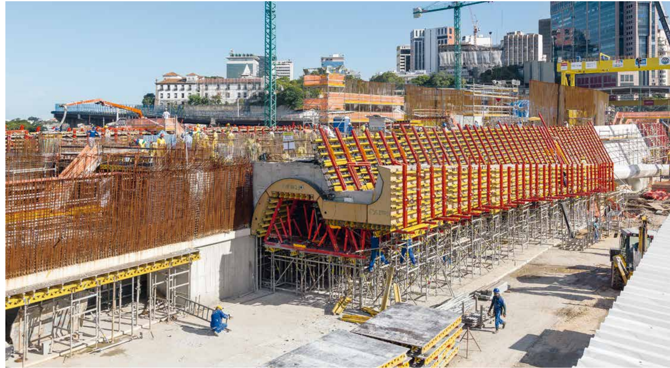
Supported by PERI UP shoring and working scaffolds, as well as a VARIOKIT raised formwork unit, the customised elements could be assembled on-site to form a complete 3D formwork construction.
