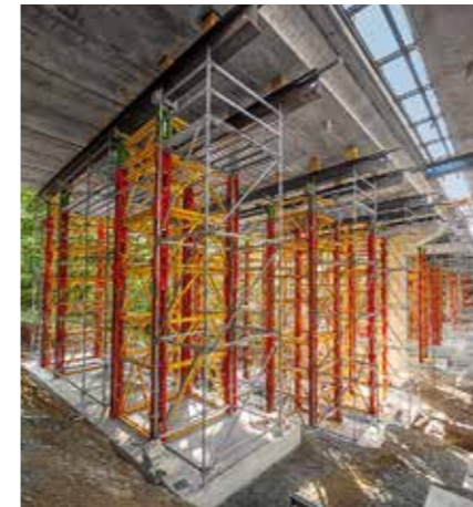
Compatible: the PERI UP Scaffolding System ensured safe access and accelerated the VARIOKIT assembly.
