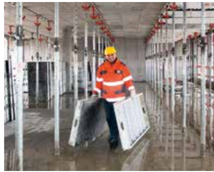
The approx. 15 kg lightweight system components support quick and simple working operations with SKYDECK.
