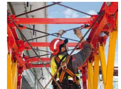
Bolted connections reduce assembly time during installation. The centric bracing connection ensures a high load-bearing capacity.
