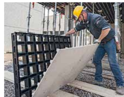
The replacement formlining can be mounted by hand using only a few screws – also on the construction site and without any special tools.
