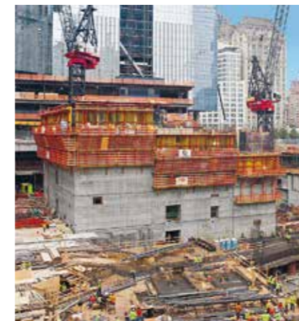
For the external walls of this 47 m x 43 m building core, the ACS R variant provides the optimum solution.
