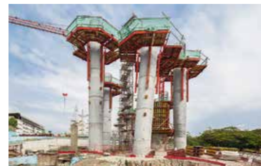
On the basis of the RCS Rail Climbing System, the inclined circular columns could be efficiently constructed.
