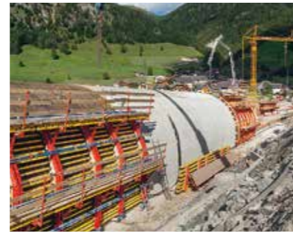
The external formwork for the tunnel arch was moved as large-sized units with the crane.
