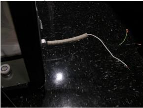
b. Cut the power line to the ballast
