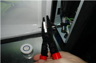
d. Connect power to the Linearray™ Driver (Black to Black, White to White, Green to ground), using waterproof wire nuts.
