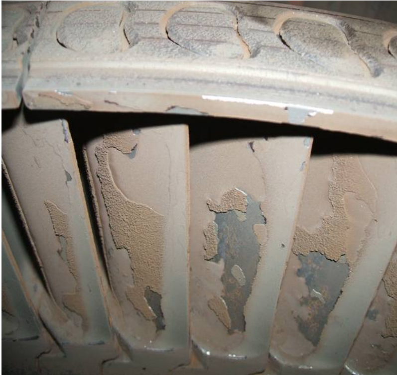
Figure 6 - Copper deposits on and HP turbine on a western US Power plant
