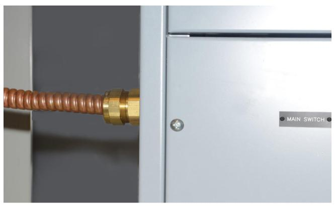
Strip armor from core and terminate to panel with readily available standard brass connector.
