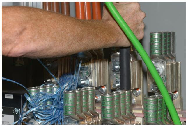
Route insulated conductor in panel and terminate without need for any splices.
