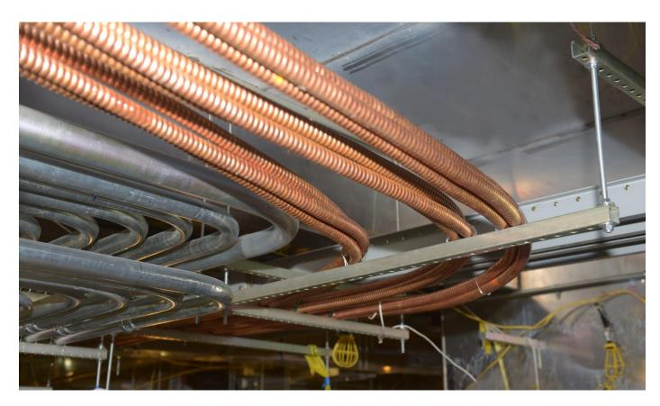
VITALink MC installs directly from reel without need for special bending equipment.
