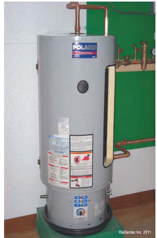
The Polaris Water Heater is all stainless steel, 95% efficient and vents through the wall or roof with plastic pipe.
