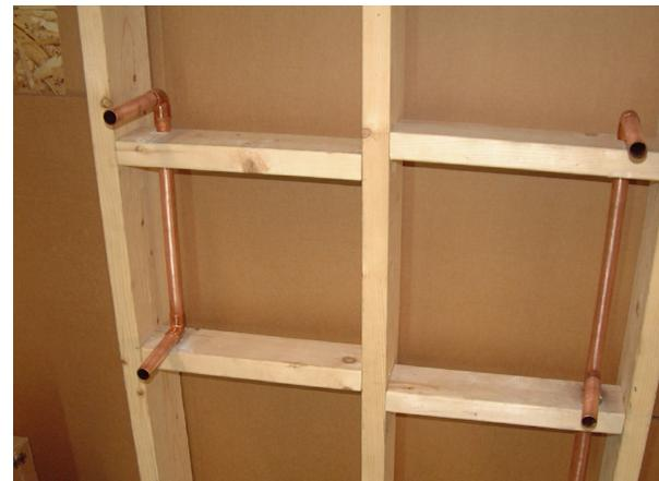
Assemble the piping and solder it together. Adjust the blocking until level and square, then fasten securely. After the sheet rockers leave, you can dress up the wall penetration with standard eustaceons. Then paint or coat with urethane.
