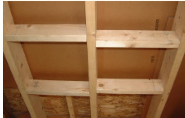
Drill the blocking where indicated and place them where they will best support the towel rack and risers. Off-set them so that you can nail or screw directly into the blocking instead of toe nailing. Don't fasten them permanently until the work is level and square.
