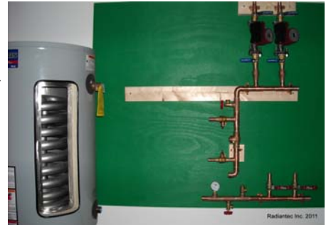
Your zone distribution manifold (ZDM) will look like this once installed.
