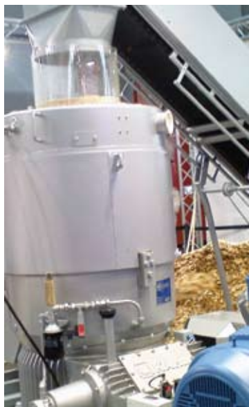
Level control of wood chips
