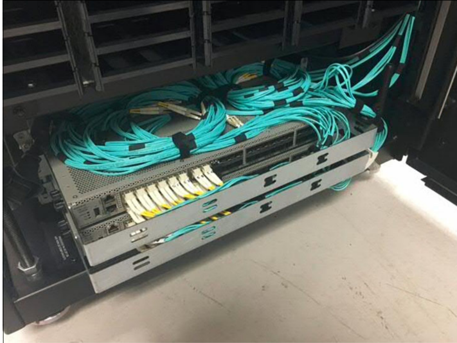
Figure 1-13 Integrated TS7700 back-end switches
