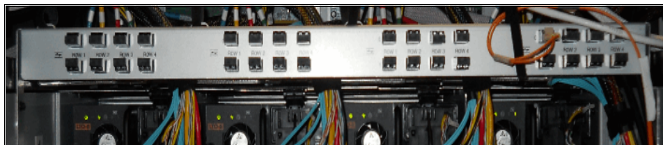
Figure 1-42 Fiber patch panel
