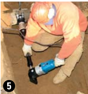
5 Make the tap, then reverse the process.
