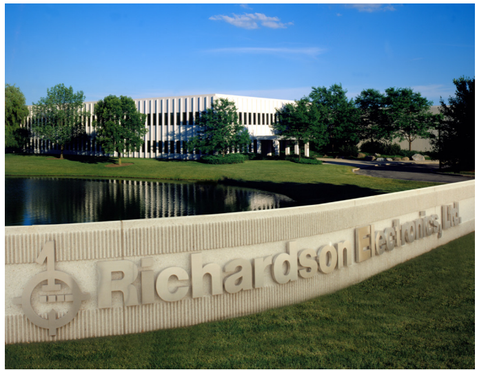
Richardson Electronics' corporate facility in LaFox, Illinois.
