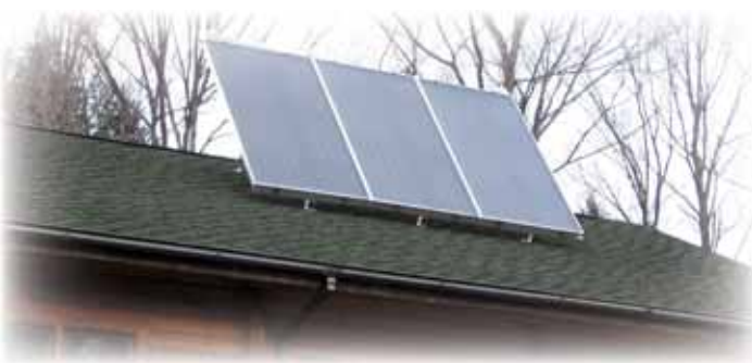
Fixed Rack Installation on a residential pitched roof
