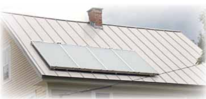
Flush Mount Installation on a residential roof
