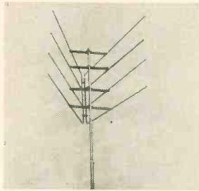
which offer complete reception on channels 2 through 83 without the necessity for couplers or double lines. The V-angle provides very directive reception on all three bands. The gain is aided by full-wave U-formed aluminum dipoles that lie vertically, forming a stacked V-angle at their juncture.
