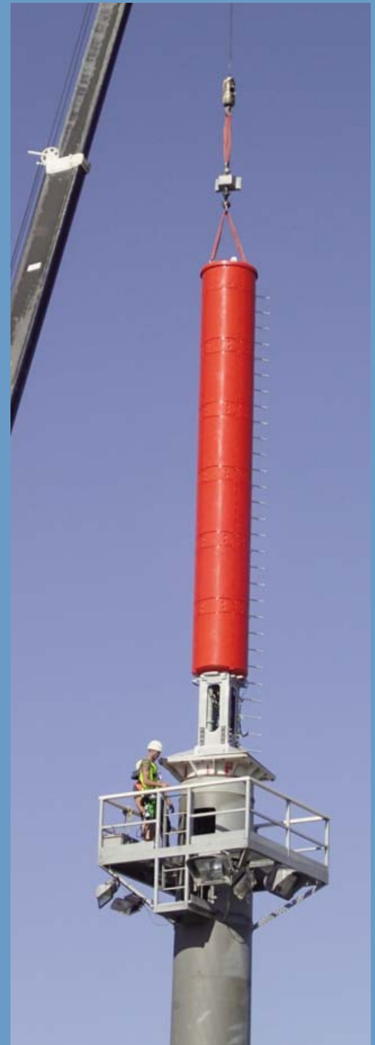
A crane has lifted the PEPL low wind load antenna onto the RFS tower in preparation for testing
