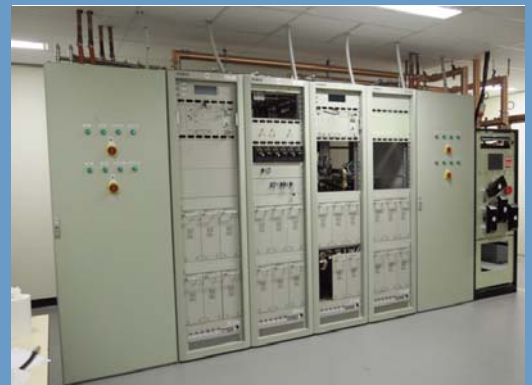
RFS UHF test transmitter
