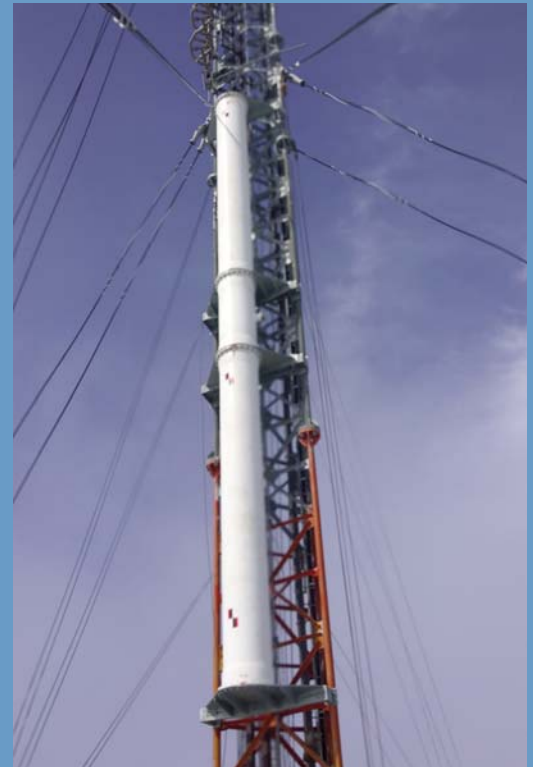
2015 RFS broadband slot antenna installed on Sutro Tower San Francisco. Photos courtesy of S. Merrill Weiss and Sutro Tower.
