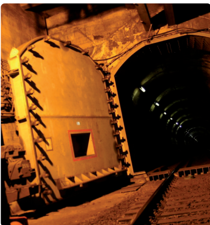
Installers had to work around the massive flood gates, which allow the tunnels to be sealed to prevent water passage during construction of highway tunnels. Existing cable sleeves were used to thread RADIAFLEX cable through the gates and into the rest of the tunnel.
