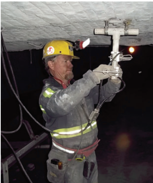
A miner installs an antenna for L-3's ACCOLADE system.
