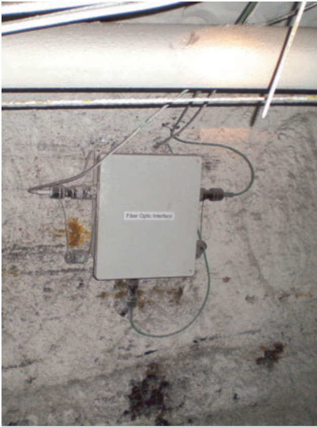
A backbone splice point mounts to the rib. (Photo Courtesy of AFL)
