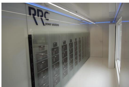
Battery Storage interior view
