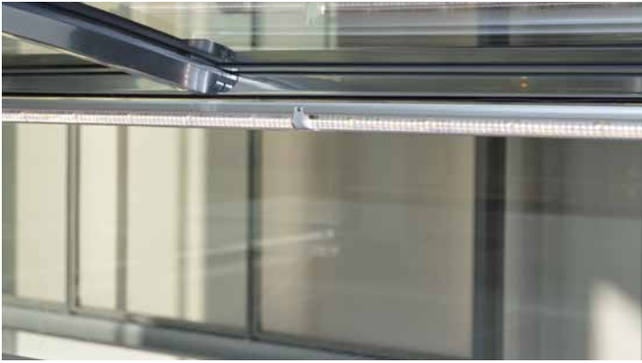
Philips LED. Placed under the handrail
