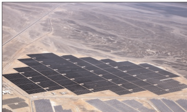
The 52.5MW Shams Ma'an Solar Power Plant.
