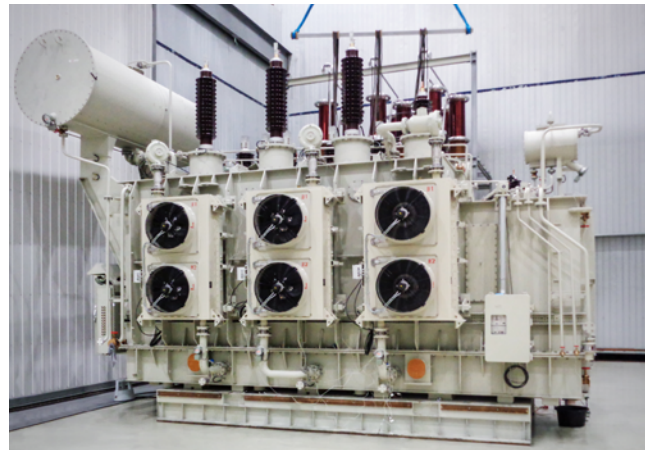
Midel-insulated 160 MVA-transformer for Moscow in the testbay at the transformer plant in Voronezh.
