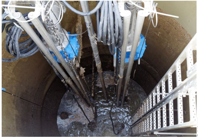
The sewage collected in the shaft is safely transported to the central treatment plant by two redundant pumps. Automation systems from Siemens transmit operational data and malfunction alerts
