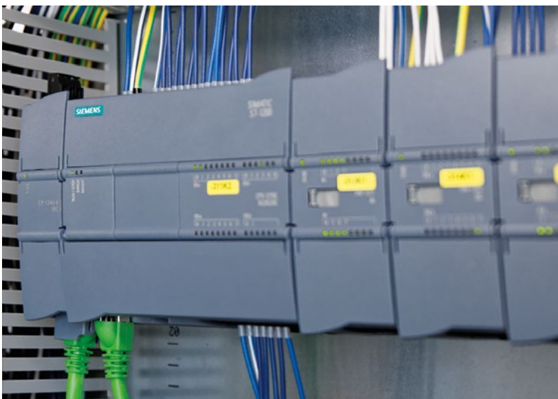
A comprehensive automation solution to help protect investments: the Simatic S7-1200 controller was seamlessly integrated into the existing telecontrol system via the CP 1243-8 IRC communications processor (far left of photo)
