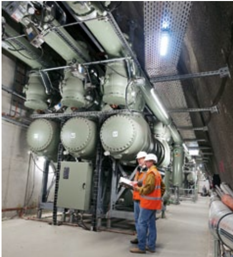
Gas-insulated transmission lines can carry high voltages in environments where masts are impractical.
