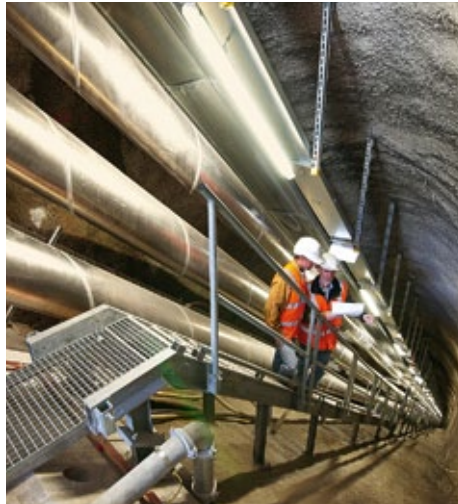
Gas-insulated transmission lines can carry high voltages in environments where masts are impractical.
